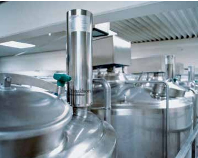
Filter housings for the aeration on storage tanks.
