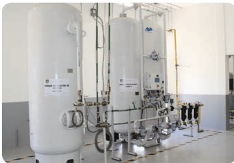
AS-Q2600-HM Duplex PSA Medical Oxygen Plant — Nicaragua
