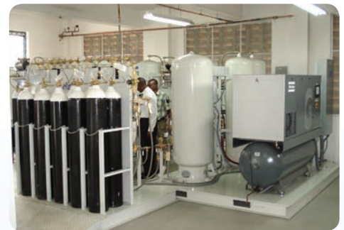
AS-J450-HMFM Duplex PSA Medical Oxygen Plant — Kenya
