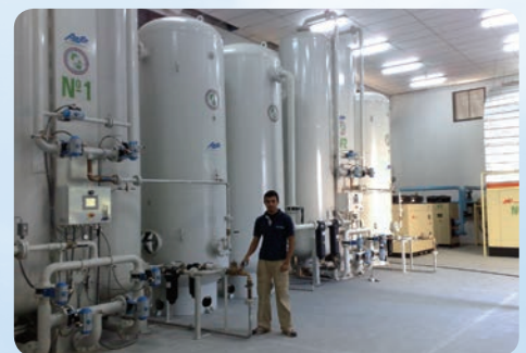
AS-Z5500-HM Duplex PSA Medical Oxygen Plant — Paraguay
